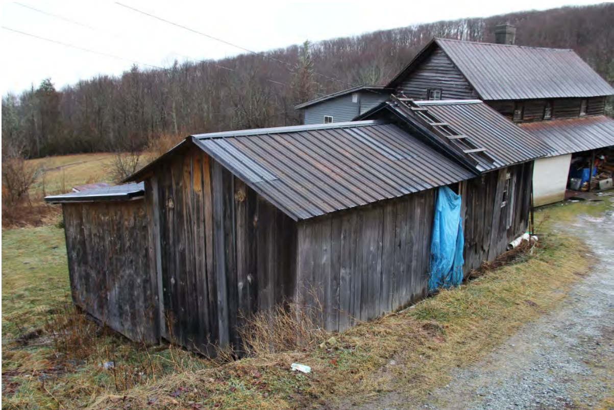
Store, oblique rear view to northeast
