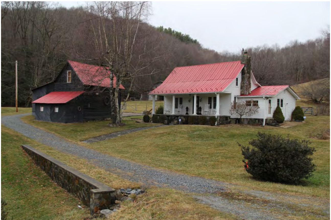
House, 273 Oliver Hill Road, ca. 1890, view to northwest
