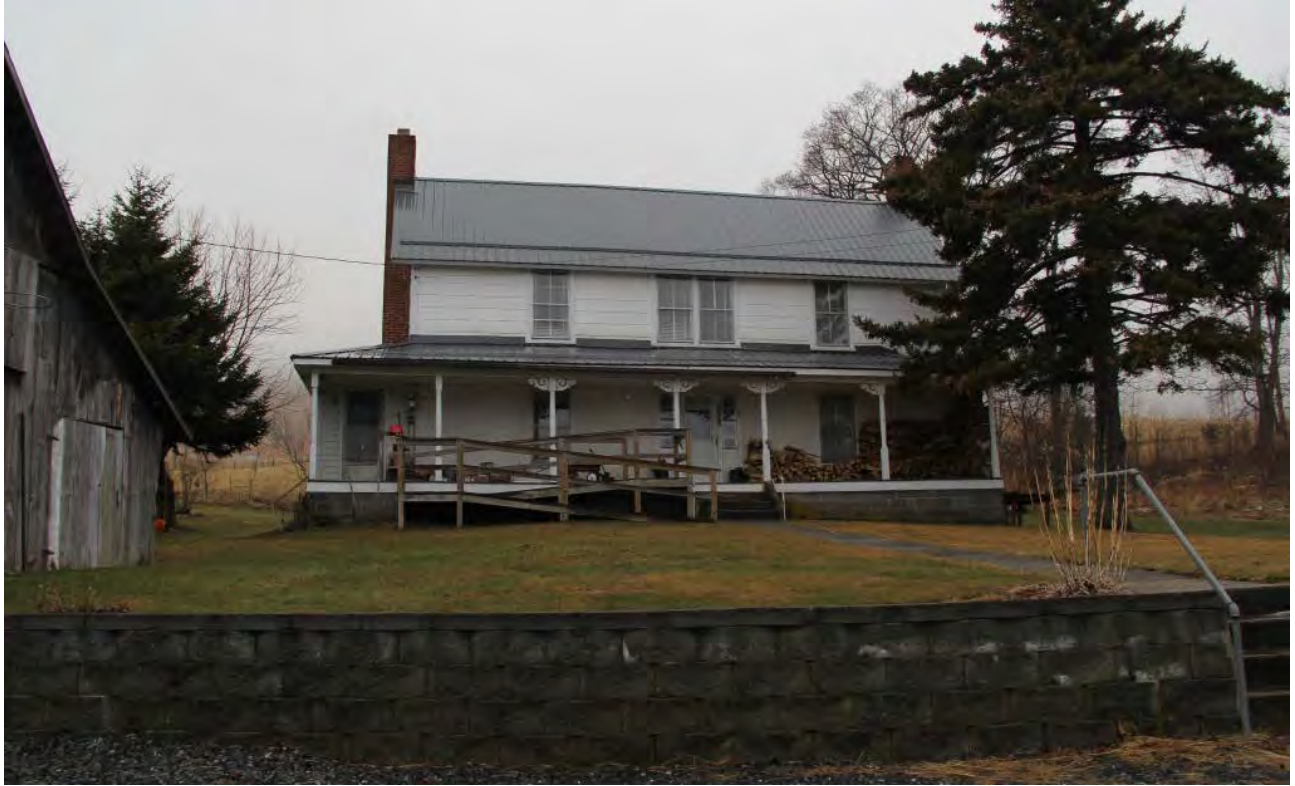
Alfred L. Yates House (WT 360), 1580 Worley Road, ca. 1880s, view to northwest
