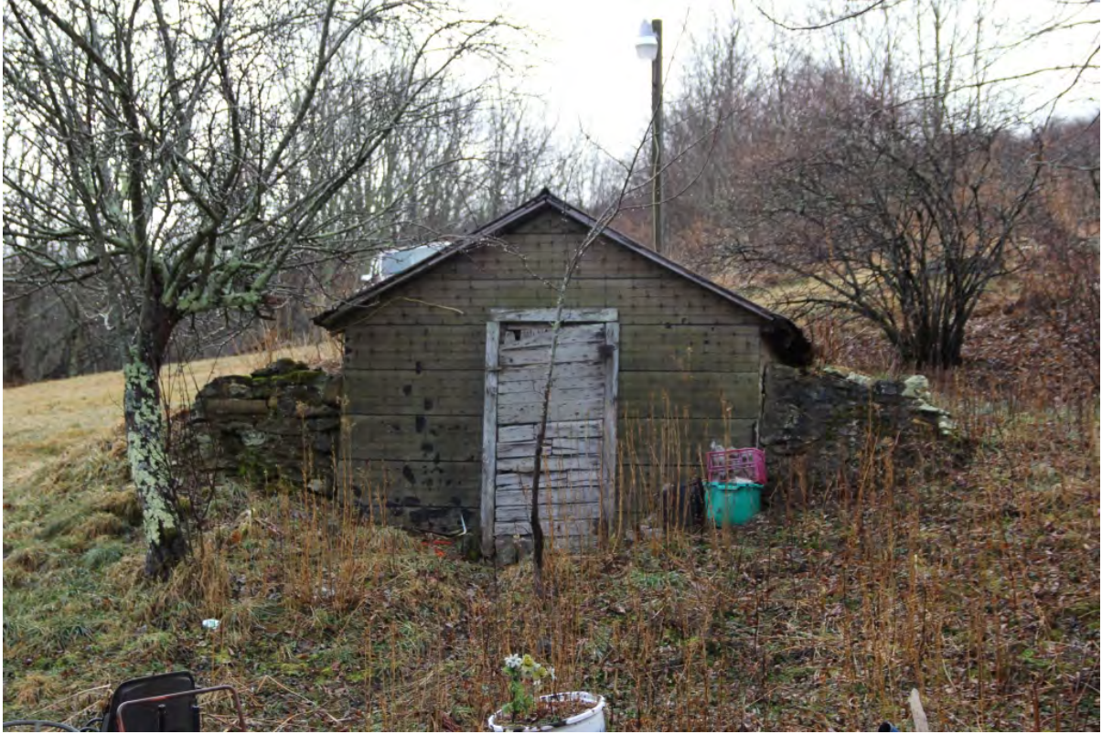
Root cellar, view to southeast
