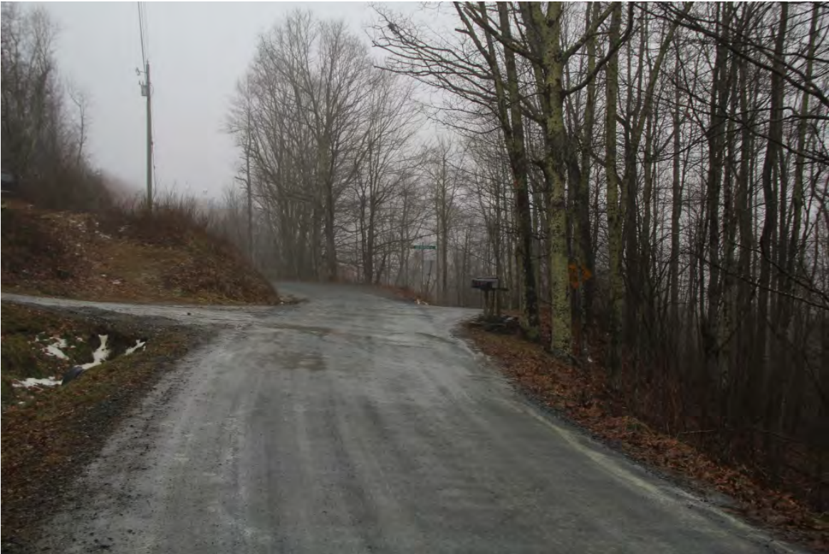
View northwest along Andy Hicks Road (SR 1128), intersection of Old Mountain Road at right
