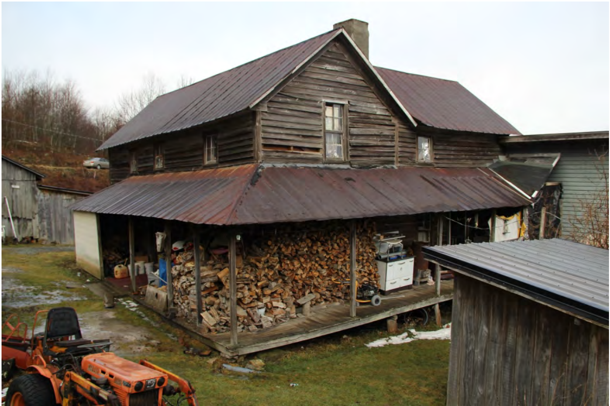
Nathan Hicks House, oblique view to northwest
