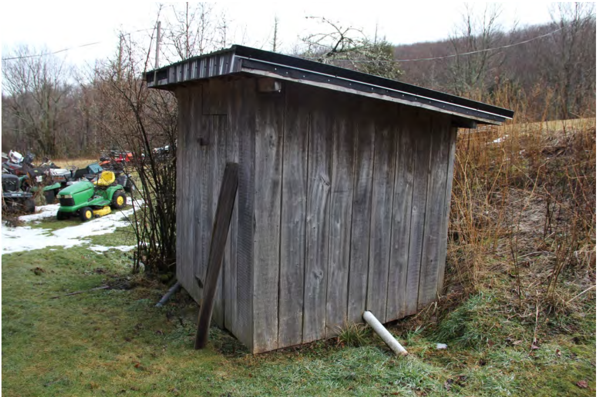
Spring House, oblique view to northeast
