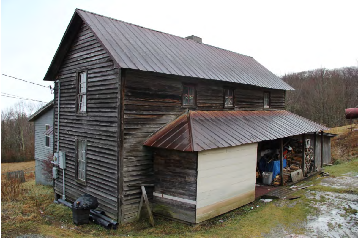
Nathan Hicks House, façade, oblique view to northeast
