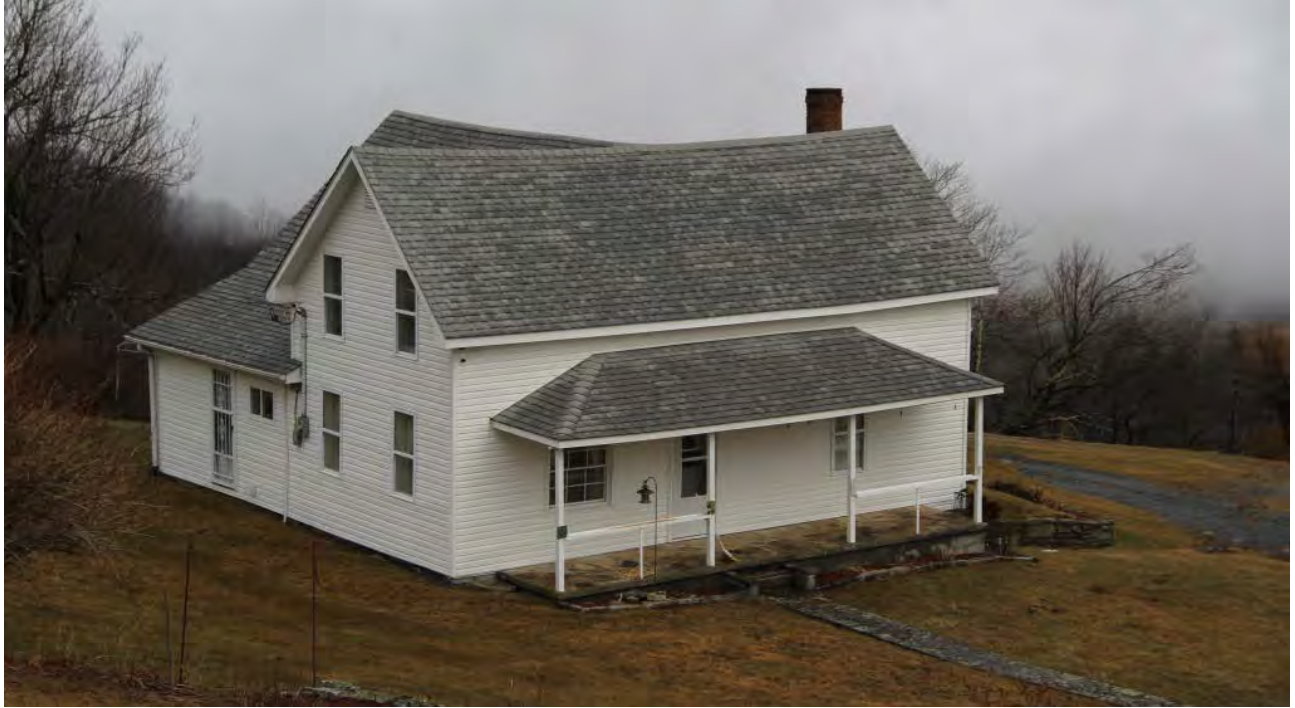
House, 5085 Andy Hicks Road, ca. 1925, view to north
