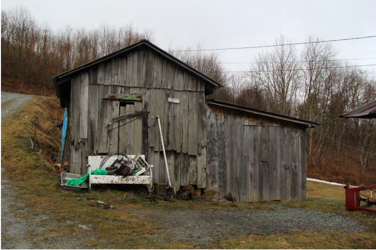
Store, east elevation, view to west
