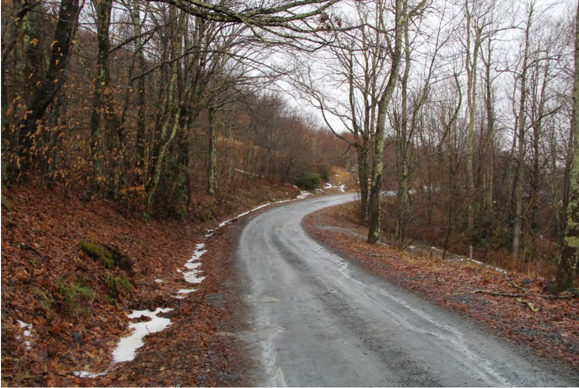
Old Mountain Road (SR 1170), view northwest from intersection with Andy Hicks Road
