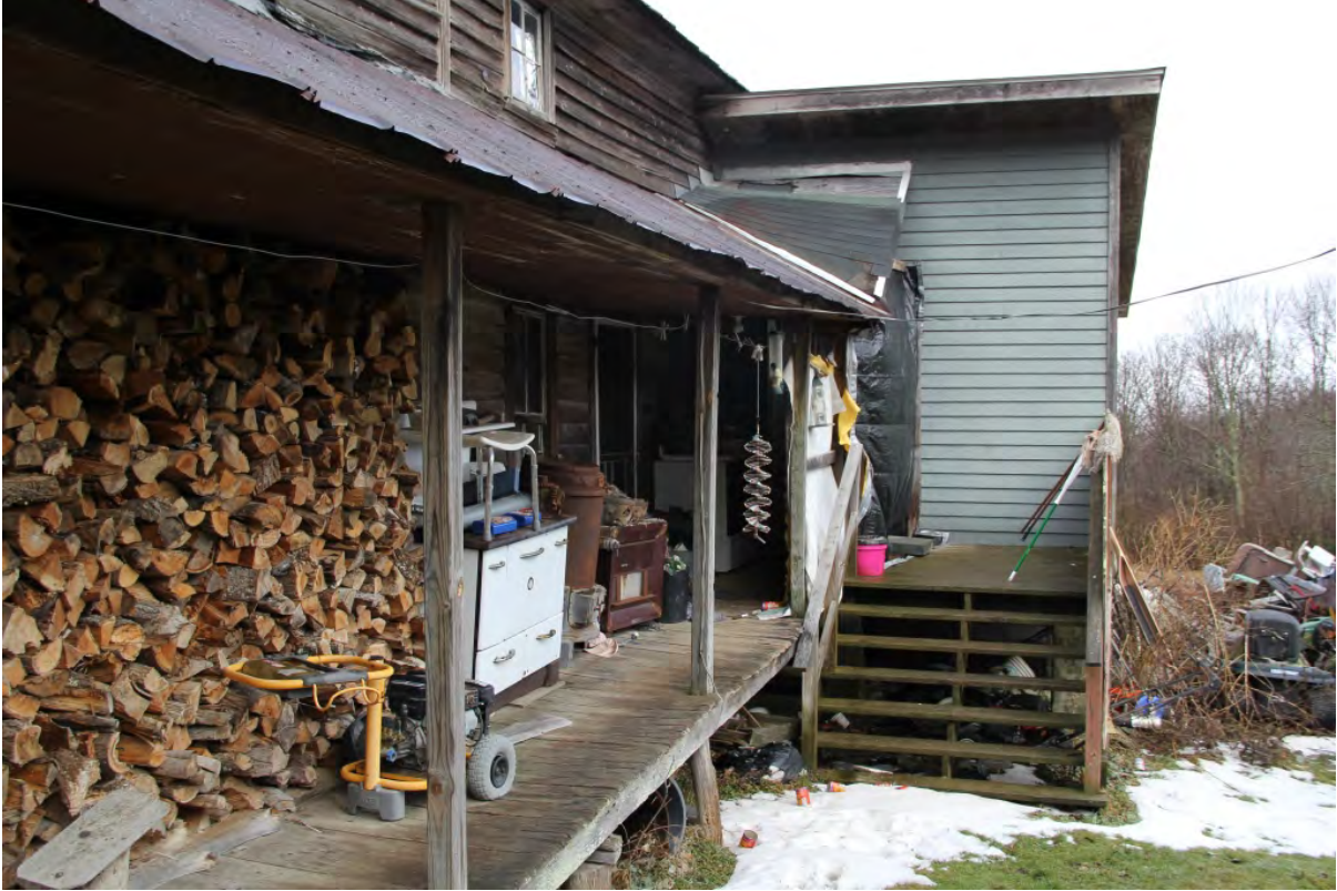
Nathan Hicks House, east side porch, view to north
